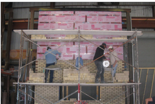
Figure 3: Test wall under construction
