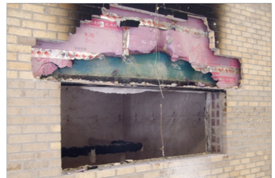
Figure 5: FOAMULAR® showing limited damage above the test window with brick veneer stripped away after the fire test
